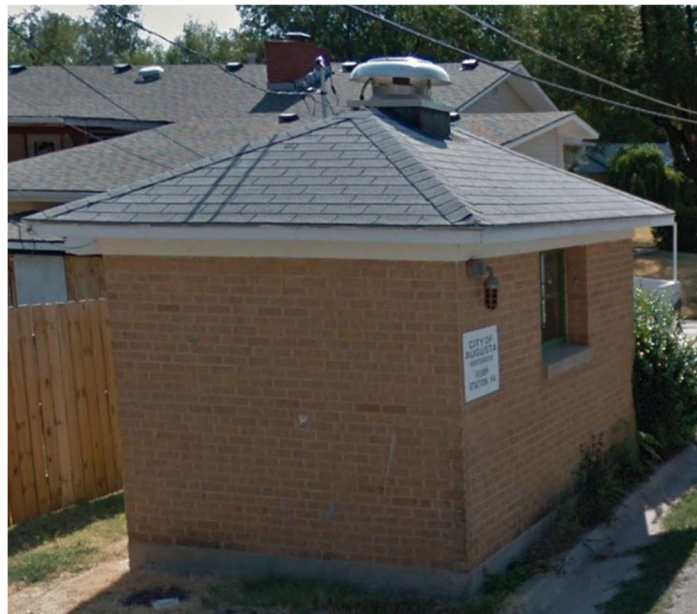
Kansas Lift Station
